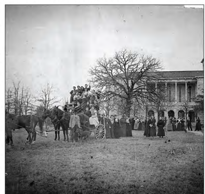
The first students and staff moved from Independence to Belton at Luther Hall in 1886. Luther Hall housed over 200 female students, along with a kitchen, dining hall, chapel, and the presidents quarters. Luther Hall burned down in January 1929.
